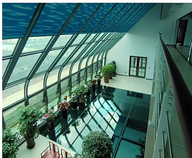
Figure 2. Light-permeable floor on the ground floor of a building with ultra-low energy consumption
