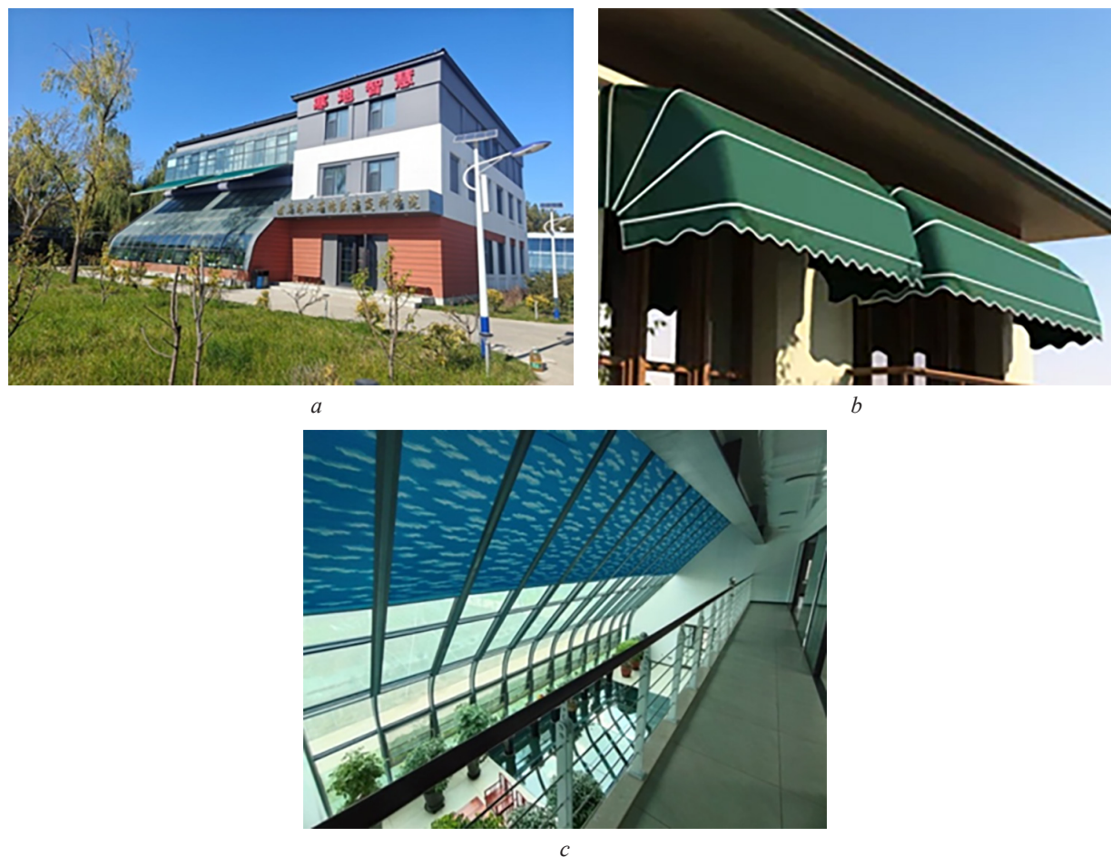
Figure 4. Examples of the use of external ( a , b ) and internal ( c ) building sun protection systems
