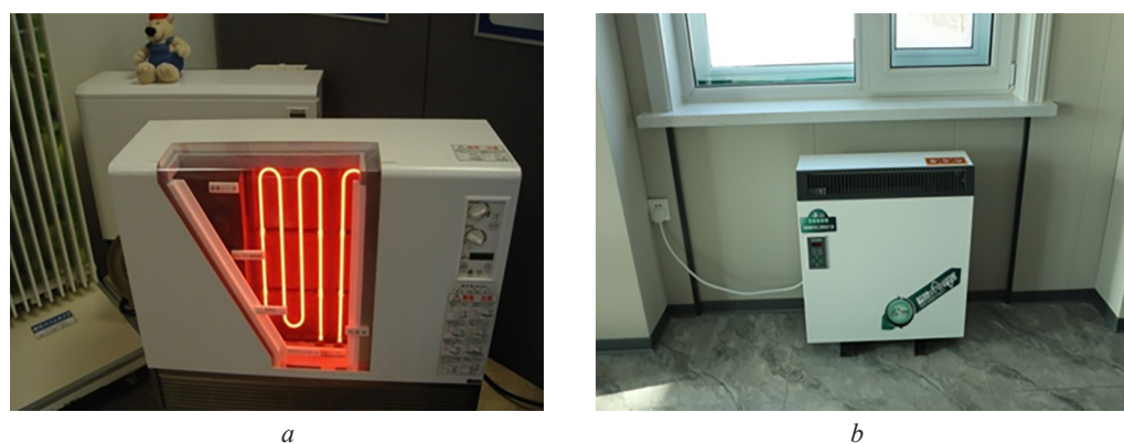
Figure 3. Operating scheme (a) and installation of an electric heat accumulator in the room (b)
